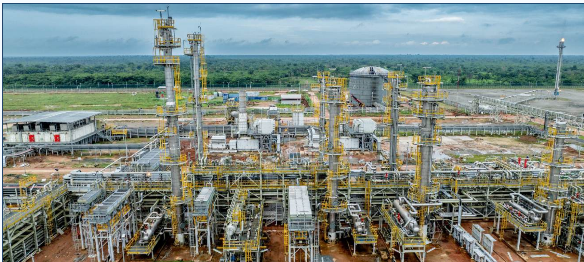
Snapshot of the 300 mmscf/d ANOH gas project
